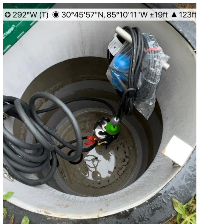
Installing grinder pumps.
