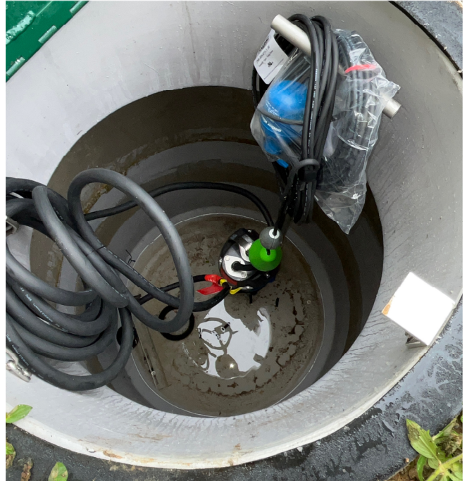
Installing grinder pumps.
