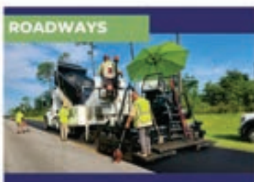
Paved and resurfaced over 14 miles of roadway.
