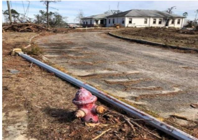
**Wastewater:** The wastewater pumping station was crushed by trees from Hurricane Michael and manholes and shallow gravity sewer lines were damaged by uprooted trees. DJJ insurances proceeds allow sufficient funds to do some wastewater manhole and sewer line repairs and repair to one pump at the pumping station to allow the relocated Sheriff's office to have wastewater service until more complete and permanent repairs can be made to the wastewater system.
