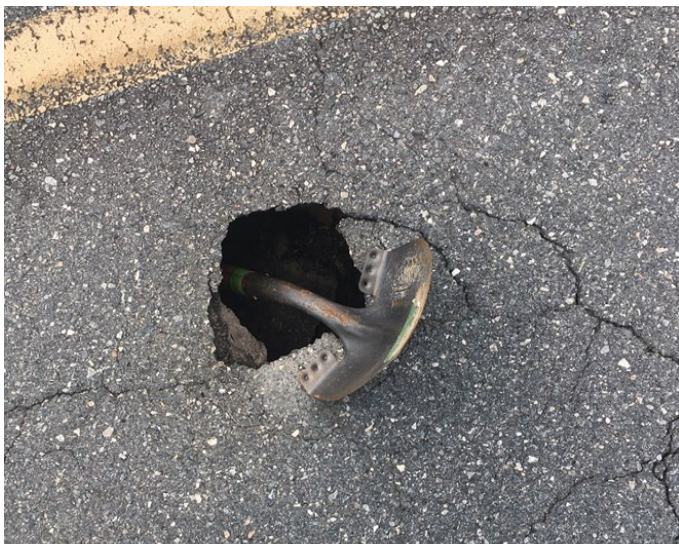
River Rd—Road damaged by beaver activities requiring emergency repairs. The shovel is used as reference to show the depth of the hole.
