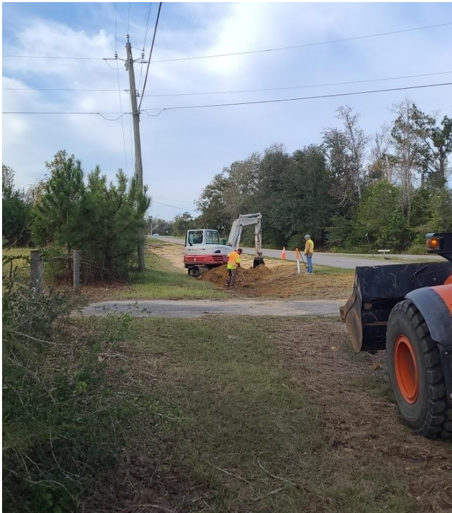
Dressing area for erosion control
