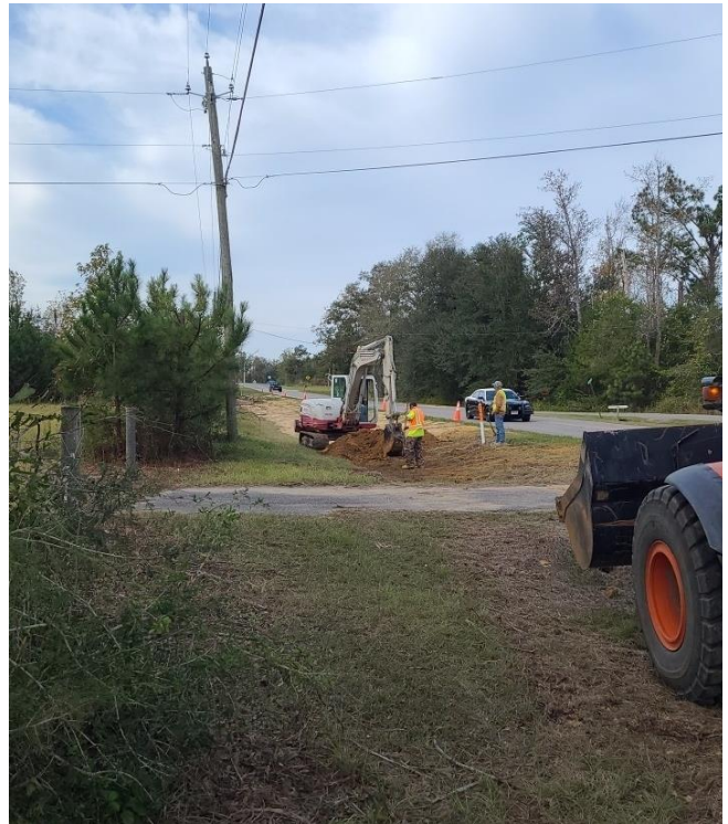
Dressing area for erosion control
