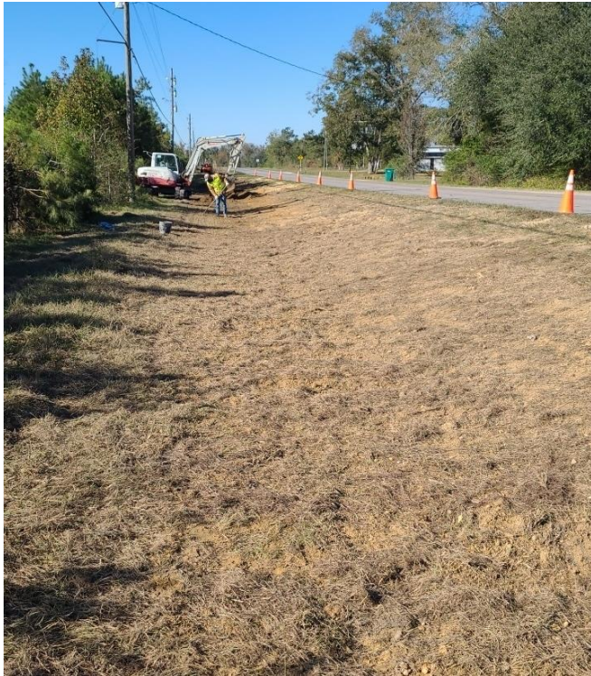
Dressing area for erosion control
