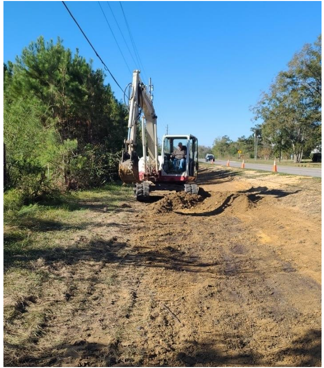
Dressing area for erosion control
