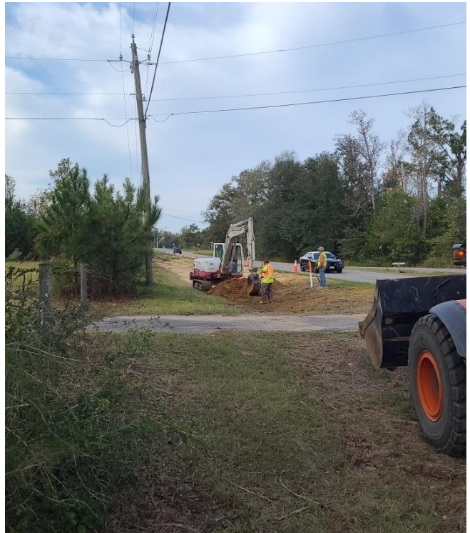
Dressing area for erosion control
