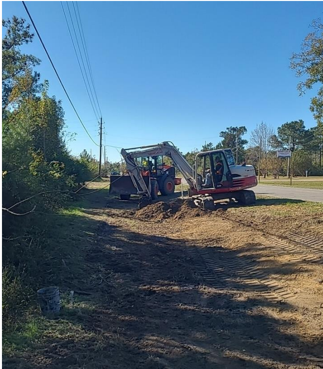
Dressing area for erosion control
