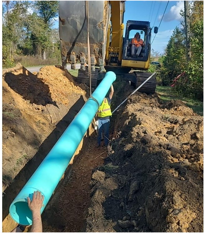
Installing force main
