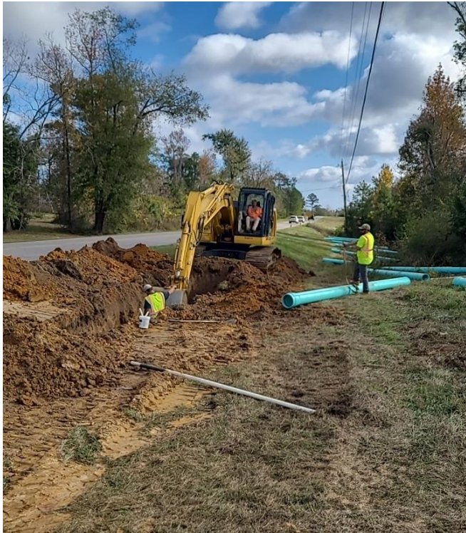
Installing force main
