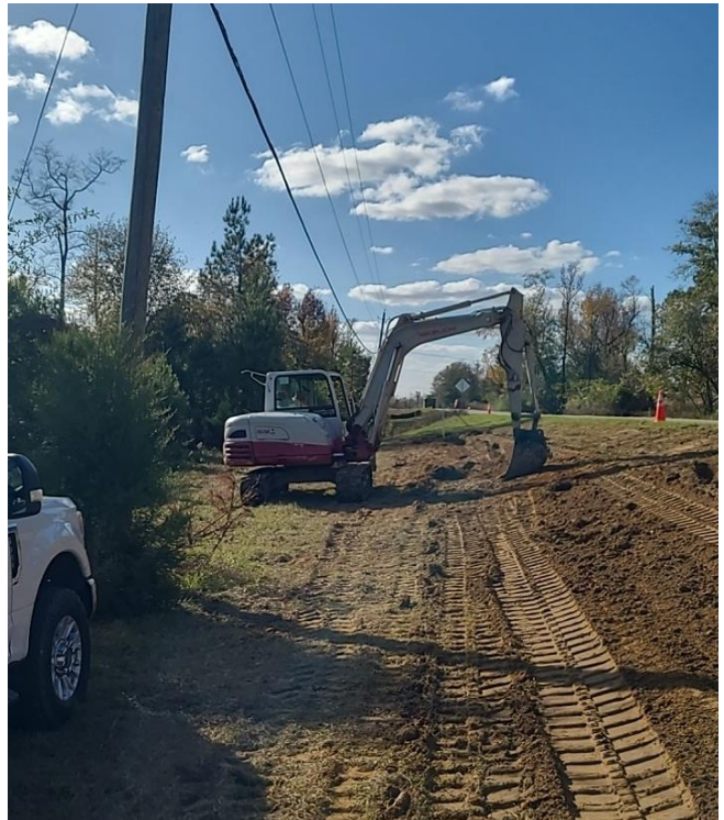
Dressing area for erosion control
