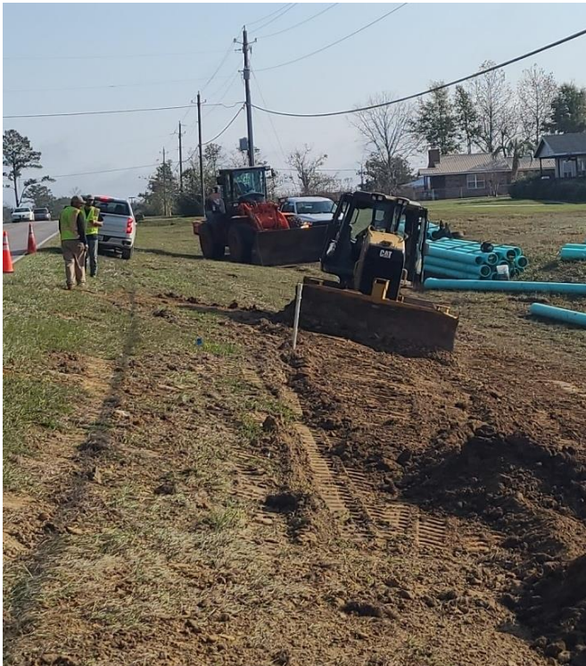
Backfilling Trench
