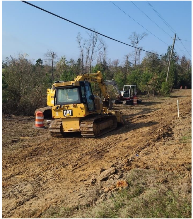
Dressing area for erosion control
