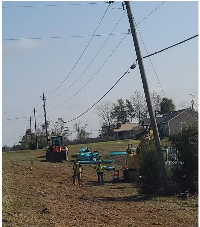
Dressing area for erosion control
