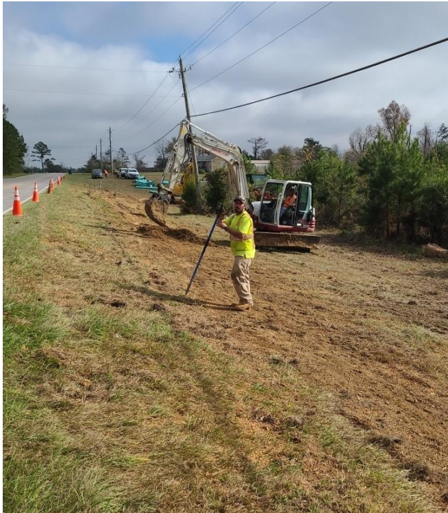
Dressing area for erosion control
