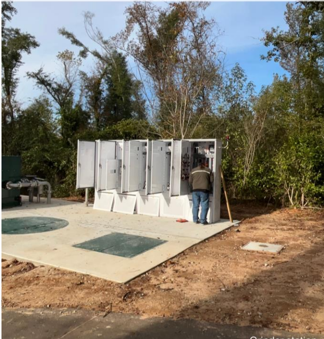
Preparing lift station for start up.
