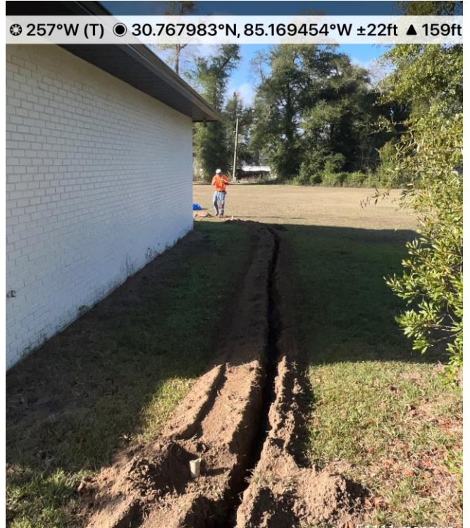
Running wires from grinder pump to control box.
