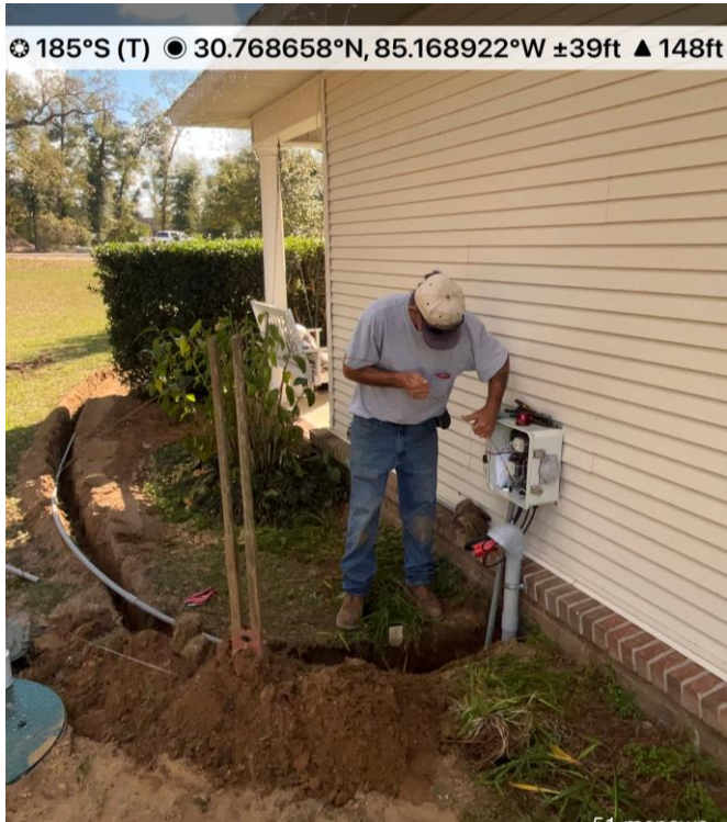
Preparing grinder station for start up.
