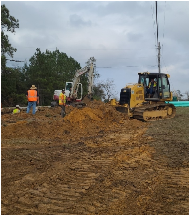
Backfilling Trench
