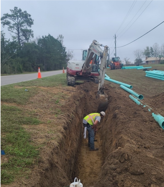
Excavating for pipe construction
