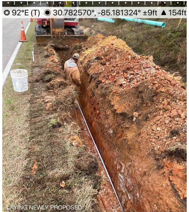
Installing 10" force main
