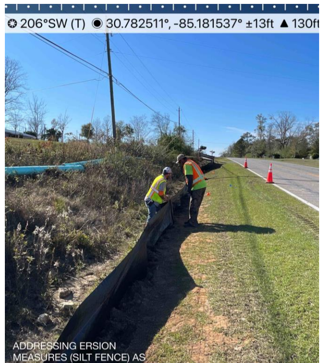
Installing erosion control
