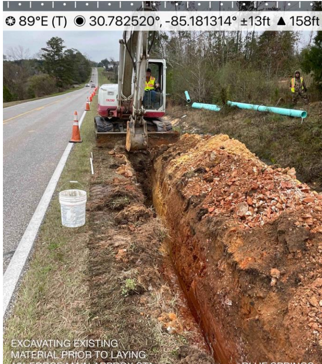
Excavating for pipe construction
