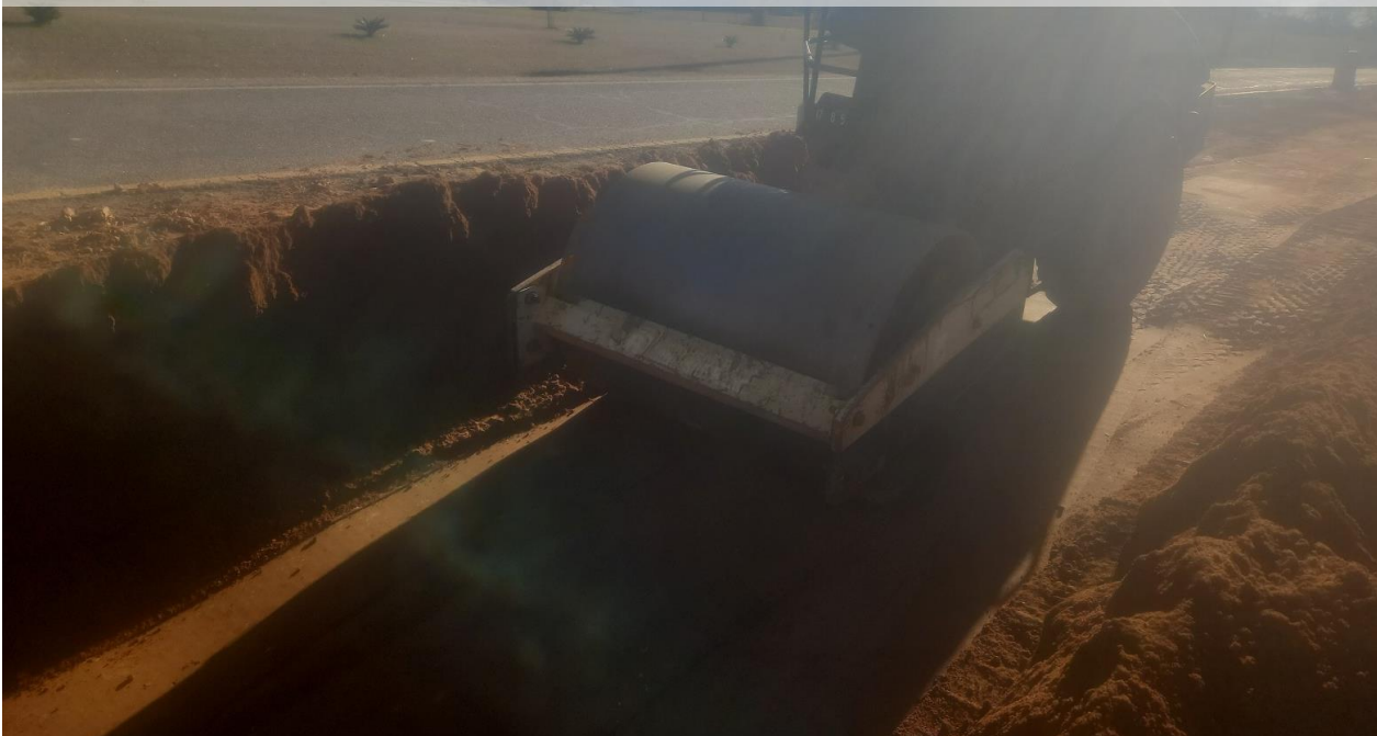
Roller packing pipe trench AHE/bhl
