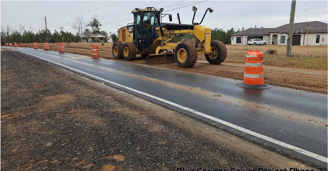
Blue Springs Sewer Project Phase 2
