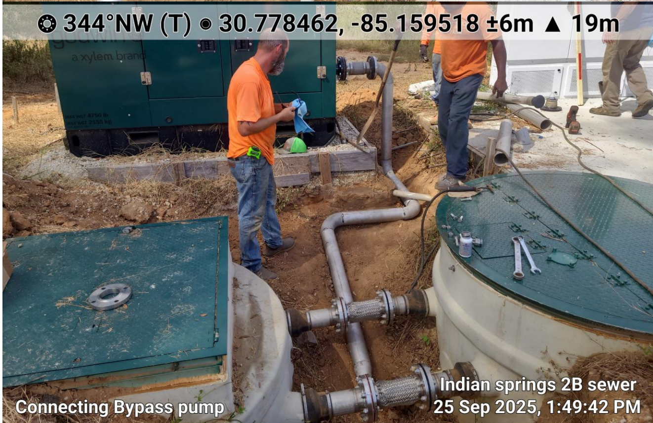
Connecting Bypass pump
